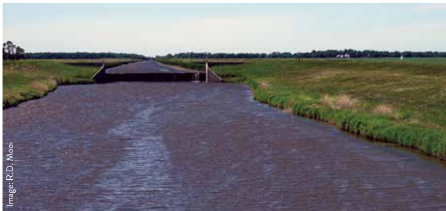
The Norquay Channel, near Carman, is a large ditch that drains a former marsh area. This permits the area to be farmed.
